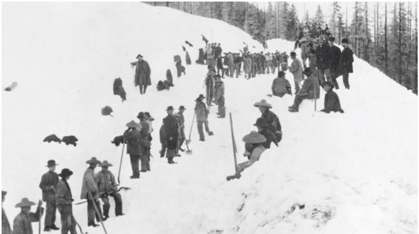
Chinese immigrant work crews prepare to excavate a snow-covered portion of the Central Pacific Railroad's route in the Sierras. (Stanford University)
